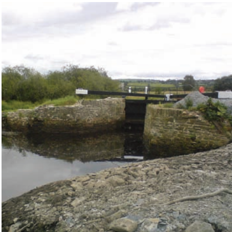
Restored Canal Lock Gates
